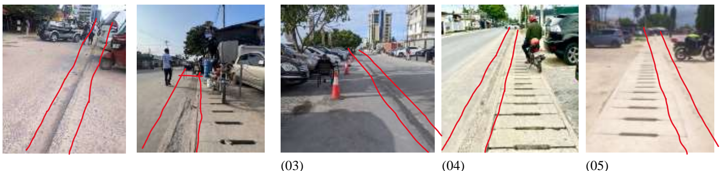
Plate 4.13: the Kerb stones removed via LGA, TARURA and TANROADS permit, to connect the semi-public spaces, pedestrian walkways and access roads, as an improvisation to accommodate car parking and a space used by imported used car vendors on Sam Nujoma service road in Sinza “A”. A far on (02) is a pedestrian walkway blocked by a retail shop. Source: Author (2024).
