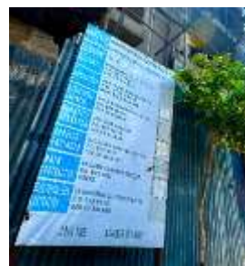
Plate 4.05: a construction of a multistorey residential apartment in Sinza "A", Source: Author (2024).
