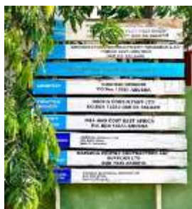
Plate 4.02: a construction of a multistorey residential apartment in Sinza "A", Source: Author (2024).
