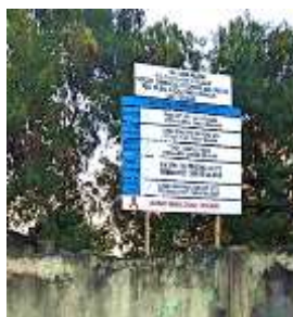
Plate 4.07: a construction of a multistorey commercial cum residential building in Sinza "A", Source: Author (2024).
